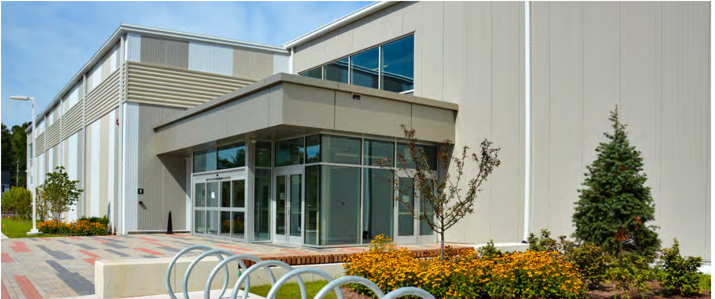
Photo courtesy of Dacon Corporation
