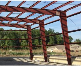
Girts and purlins attached to primary structural steel frames. Various types of bracing shown, such as xbracing, flange bracing, girt/purlin bracing.
